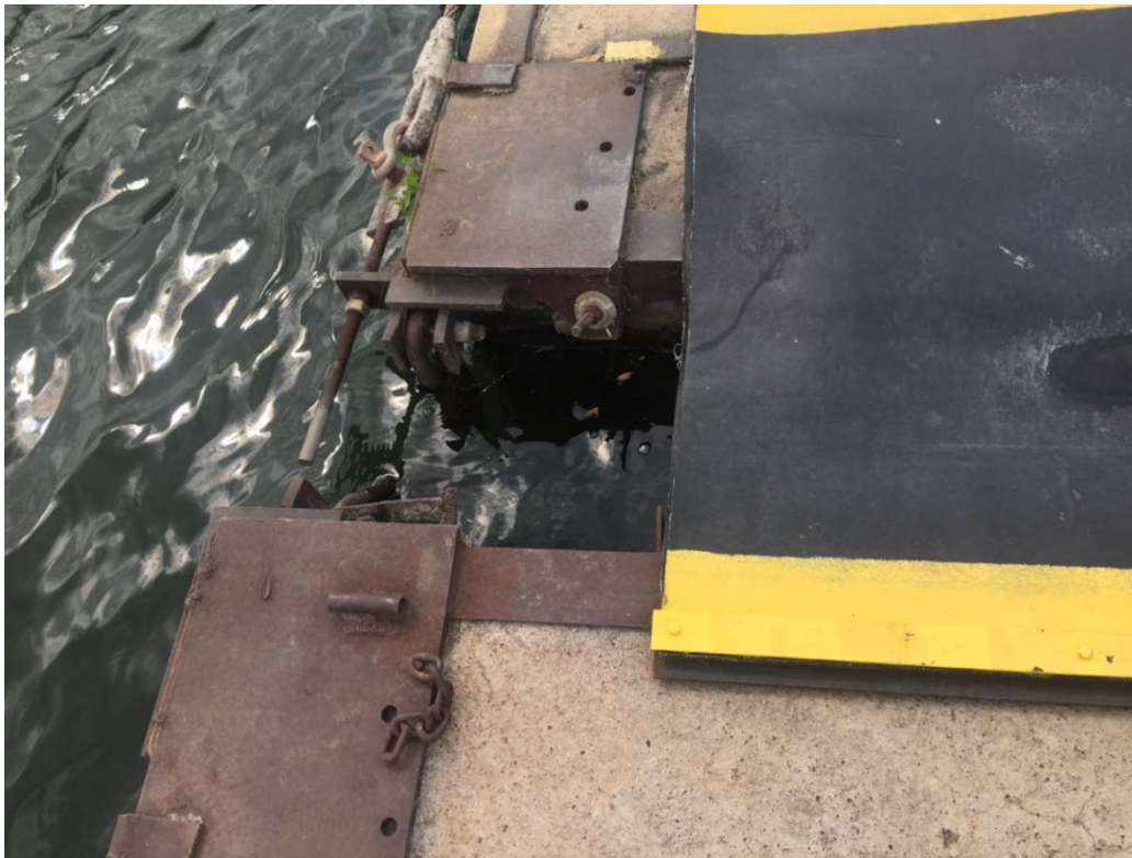
Figure 16. Breakwater Section Hinge Assembly
