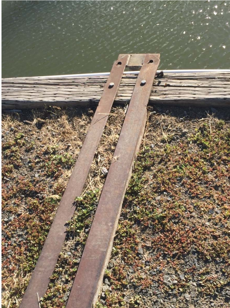
Figure 19. Bulkhead Steel Strap Repair
